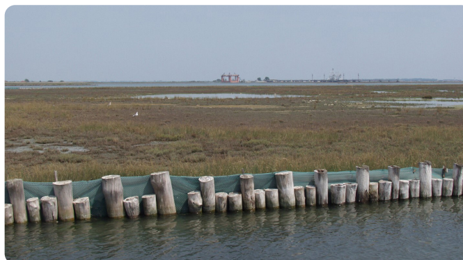
Piling technique to protect salt marsh edges
